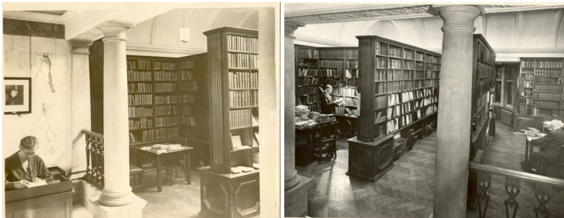
The BDA library after its removal to Hill Street
